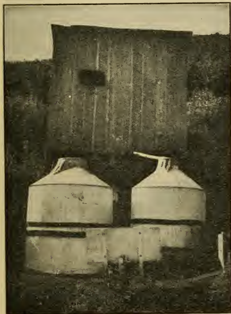
Typical sidehill California honey-house. The honey runs by gravity from the extractor thru pipes into the large tanks located below the building on the outside.
